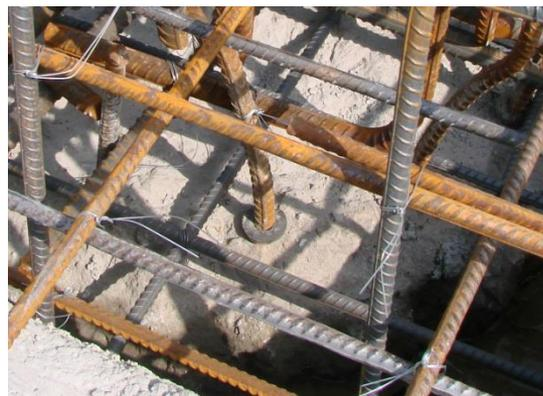
桩头受力钢筋根部应采用遇水膨胀止水条
